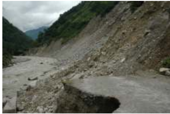
Figure 19: Ghingrani Landslide near Shilling, with little evidence that there was a road here before
