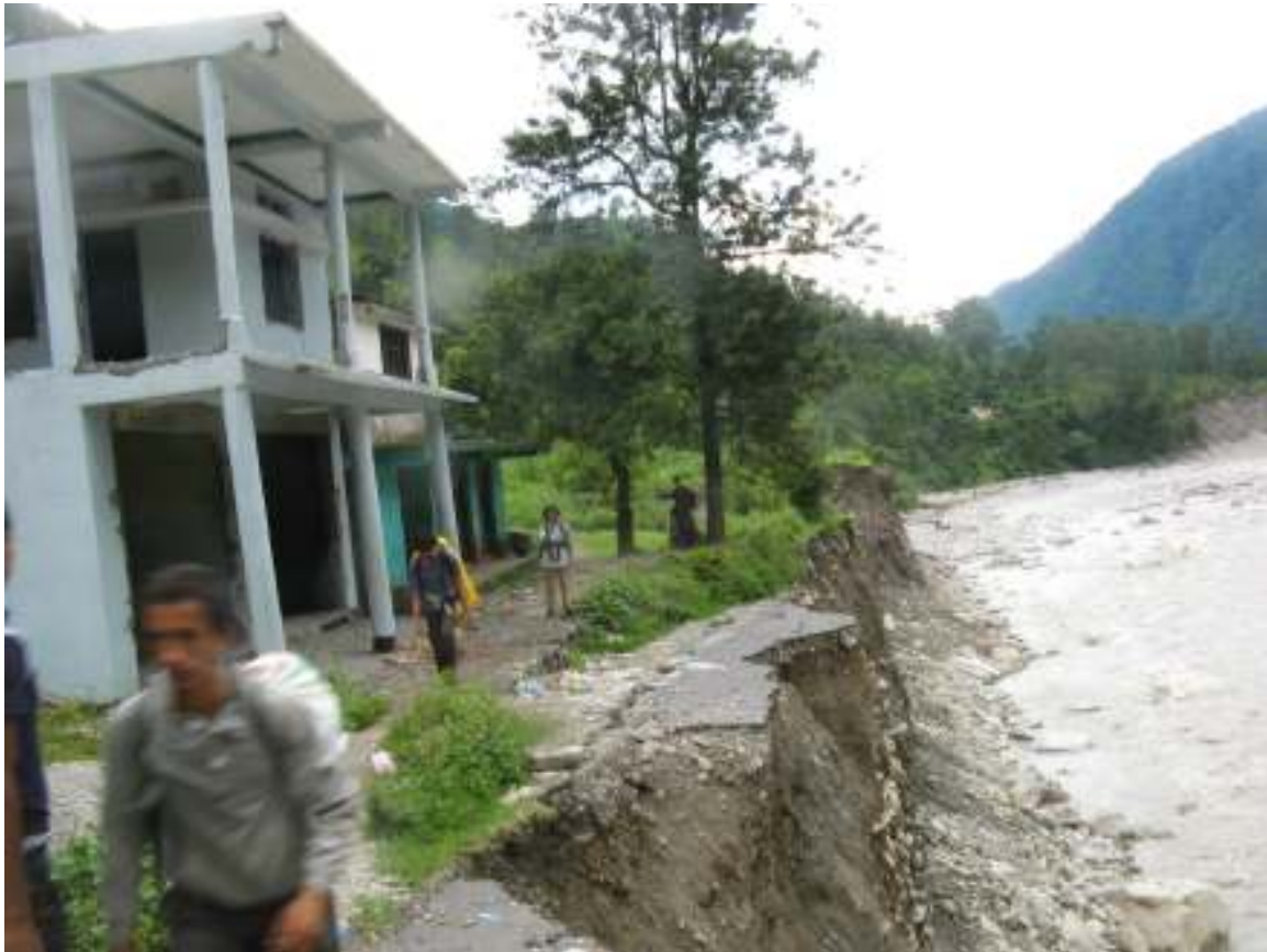
Figure 14: Lumti Village - Abandoned shops and homes, the habitation that existed on the right side of the road has been totally destroyed in the floods
