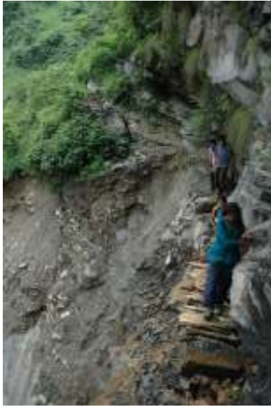
Figure 18: temporary and dangerous path between Khinwagaon and Umargada
