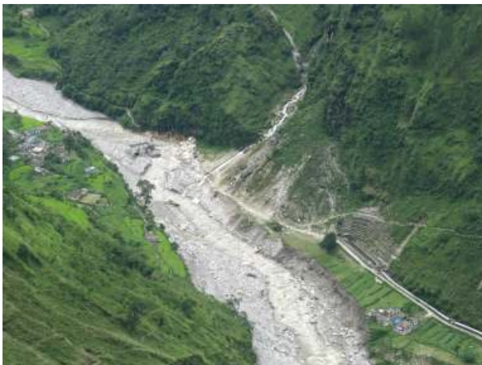
Figure 20: View of the Paina River, a tributary of the Gori. Visible are – Centre Left - the destroyed barrage of the 5 MW Motighat Hydro Project, Right – Washed away farms and precarious homes of Lodi Bagad hamlet and Left Dani Bagad Hamlet
