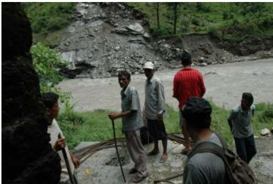
Figure 11: Mankot Rope trolley (2013) - After the flood; again note that the section that has given way is almost co-terminus with the road building induced damage. The abutment on the opposite side has caved in and has been swept away.
