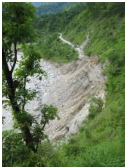
Figure 12: The new landslide at Toli, which is the current road head location
