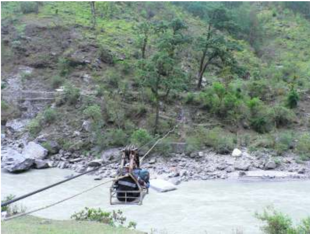
Figure 10: Mankot rope trolley (2008) - Note the structural damage to the opposite slope on the left. People in the village said that the landslide happened when road building was undertaken in the early 80's
